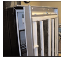
4. Remove the existing face panel, by sliding it up and out of the door surround.
